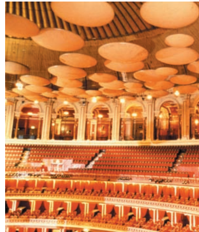
FIGURE 20.8 The plastic plates above the orchestra reflect both light and sound. Adjusting them is quite simple: What you see is what you hear.
