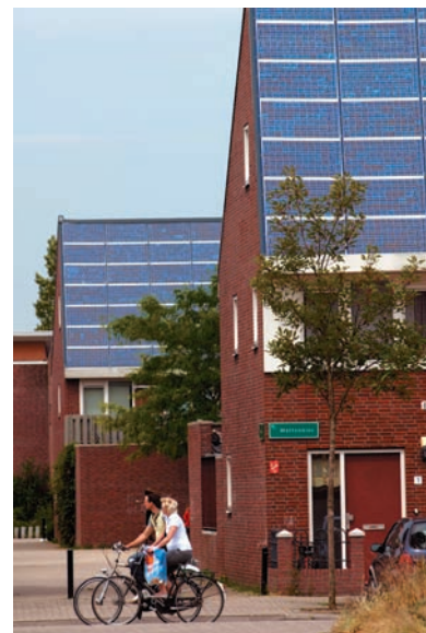
FIGURE 7.25 Photovoltaic solar cells on more and more rooftops (and sides of homes such as these in Holland) absorb sunlight and convert it to electric energy.
